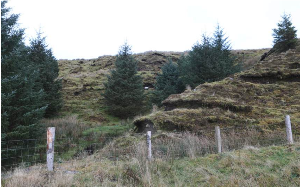
Clear Land Slippage above Coillte Plantation 7th December 2022 (Joe Sheeran) (54.328736638888884, -8.114504999999996)
